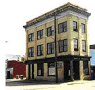
Bank of Robersonville, Robersonville, NC
